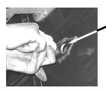
APPLY SUPPLIED SILICONE AROUND AND IN ALL MOUNTING HOLES FOR THE BRACKET
